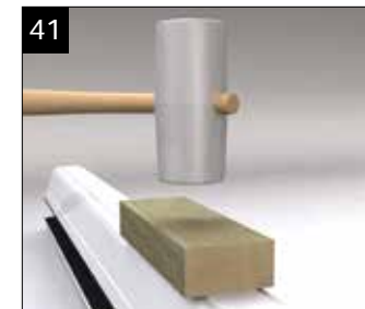
Knock the glazing bar top cappings on with a Deadblow hammer. Greater care is needed in cold weather. Keep all trims wrapped while fitting for protection.
