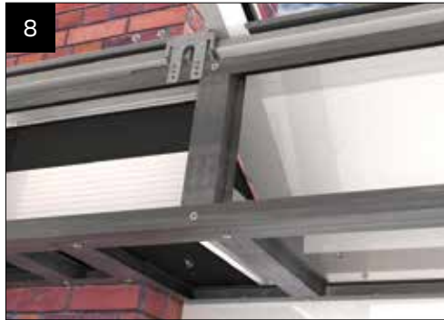
Fix the vertical frames in place using CHA006 (bag of 25) as per standard installation.
