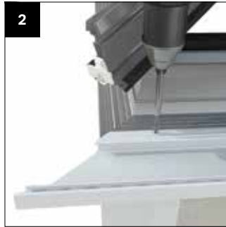
Remove the under gutter trim and dispose of it. Prior to fitting gutter offer up the lower Cornice section then secure into position using the fixings provided (CRN007). Please note: Always start with the front facet!
