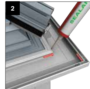
Silicone seal front and back edge of lower Cornice sections (be generous). Similarly butter 'DAM' sealer - position within 50mm of any stop end or outlet.
