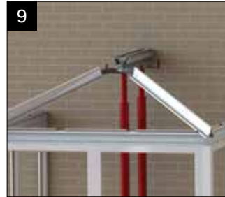
Locate the hip onto the bolts at the eaves. Loosely secure with flanged nuts. Repeat these steps until all hip and intermediate bars that meet the spider, have been positioned.
