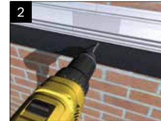
Drill through the top edge of the aluminium box gutter at 600mm centres. A fixing must be positioned within 50mm each side of the joint. Offer second half of the box gutter up to the internal sleeve and push firmly on. Fasten this second box gutter run to the host wall with masonry anchors suitable to the substrate. Ensure both sections are level and flush.
