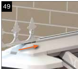
49 If cresting is specified, insert the cresting down the channel on the ridge top cap. This may require trimming to suit.
