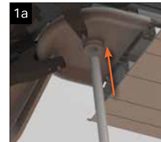
1a Tie bar at finial Insert the tie steel rod thread into the base of the spider. Measure the drop of the rod and cut to suit the position of the tie bar boss ring.
