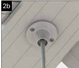
Thread the tie bar rod into the ridge fixing cover. Measure the drop of the rod and cut to suit the position or the tie bar boss ring.
