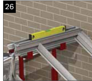
Ensure the ridge is level.
