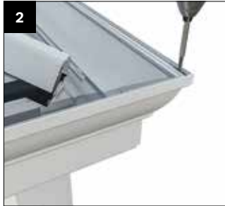
2 Secure the corners using the cleat (CRN001) and fixings (CRN006).
