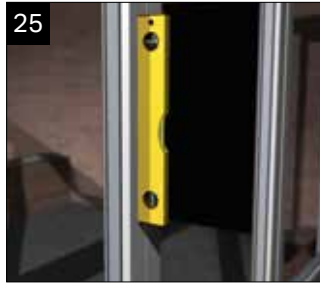
Check the window frames are plumb.
