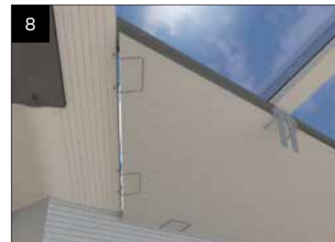
8 Attach the cloaking panels and fit as shown in the main pelmet installation guide. (page 16).
