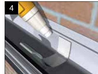
Check surfaces are dry, clean and grease free. De-grease if necessary. Heat both the sealing tape and the box gutter with a heat gun and position the tape over the joint. Press the tape firmly across the joint of the sleeve and the box gutter ensuring there are no air pockets.
