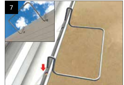
7 Refit the clips with the clip leg extending through the holes.
