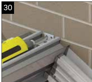
Drill through the holes on the ridge fixing bracket and secure with the correct masonry anchor. Now fasten the frames to the host wall and the dwarf wall.
