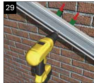
Drill the starter bars/masonry within 200mm of the ridge and eaves beam plus at least one more equidistant between the two. Pack out to support the starter bar behind each fixing before fitting the correct masonry anchor.
