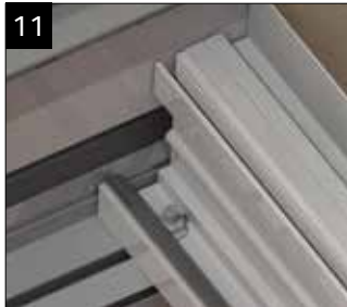
Secure with flanged nuts at ridge and eaves.
