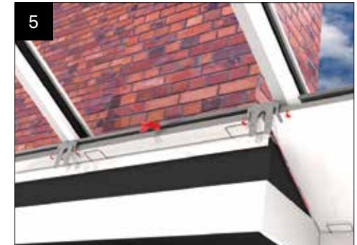
5 Fit the polycarbonate modesty panels and bend over bracket legs to secure.
