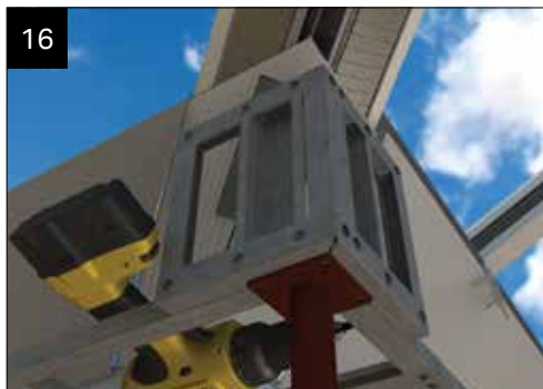
16 Valley infill panel fitted to horizontal frame, as image 10.
