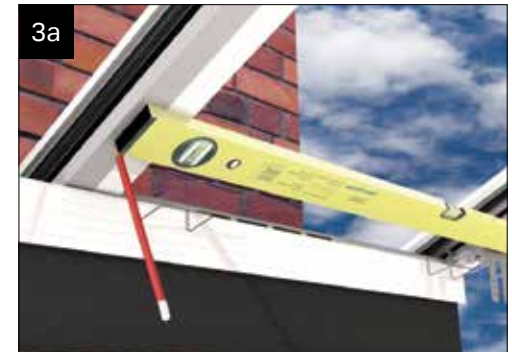
3a FITTER TIP: If possible, check and line through with the bracket position on the adjacent full length bar. Mark the bracket positions on the bars off the box gutter.
