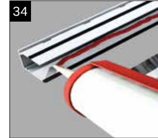
Take the glazing end profile and run continuous bead of sealant (appropriate for glazing) immediately behind the co-extruded gasket (along the full length). Now seal the space between the glazing end profile and the sealed unit (see inset) at each end (DO NOT DO THIS ON POLY ROOFS).
