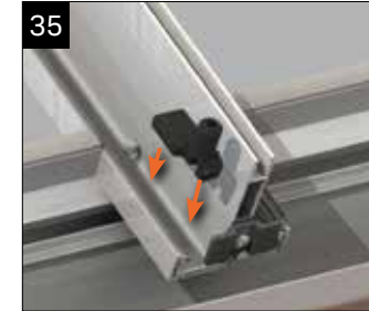
Snap off appropriate handed glazing stop. Place this into the base of the glazing bar.
