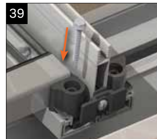
Ensure the glazing stop is pressed tightly up against the end profile. When in position use the fixings provided to fix the glazing stop down into the bar as shown. Ensure clip offers maximum support to glazing at all times.
