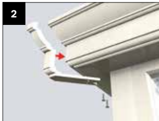
2 Whilst ensuring that the corner remains located in position, screw fix using self drilling screws CRN007
