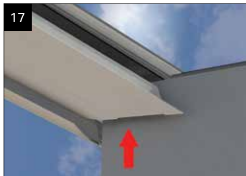
17 Valley cladding being fitted against pelmet. After plasterboard and skim.
