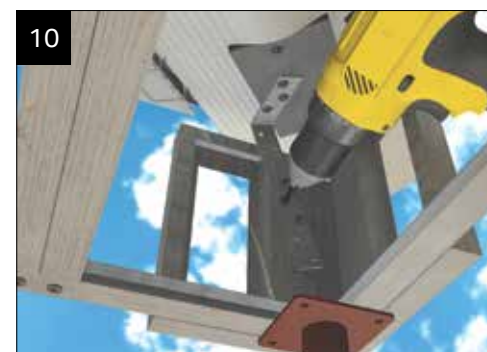
10 FIT THE STRAP CHA018 USING M4x13 SELF DRILL SCREWS, to the valley corner infill panel and the valley fixing plate. It may be necessary to bend CHA008 to suit.
