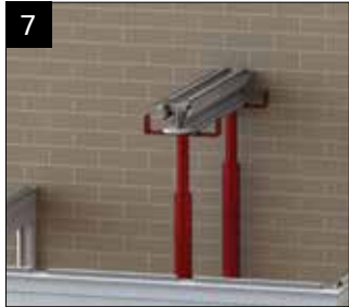
Support the ridge at the host wall and crown point. Ensure the spider has been pre drilled, glazing fascia and glazing pocket have been fitted. Fitters Tip: Pre-stress the ridge by supporting it 10mm higher than specified at the crown point.
