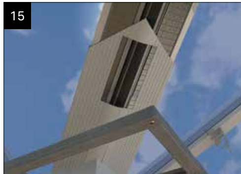
15 Fit the valley plate CHA016 (refer to steps 1-5, valley standard)
