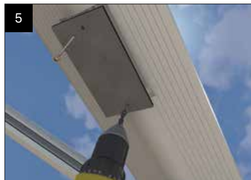
5 Fit valley plate as shown to the valley wing central connector using CHA017 (2x4.8x70 self tapping screws).
