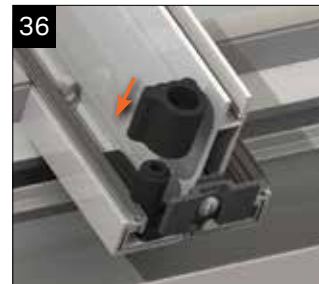
Snap off a grommet from the kit, this will slot over the upstand on the glazing stop. Repeat steps 35 & 36 for all glazing bars on the roof.
