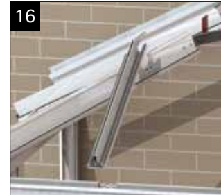
Offer up the jack rafter on to the hip and locate on the bolts at the eaves. The jack rafter bracket should be angled towards the specified hip
