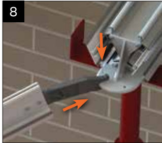
Offer up the first hip bar to the spider, insert the location pin through the spider arm fixed to the hip. Locate the pin into the pre drilled relevant hole on the spider.
