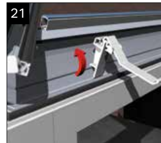
Fit all the gutter brackets supplied with the kit at maximum 750mm centres and maximum 200mm from each corner.
