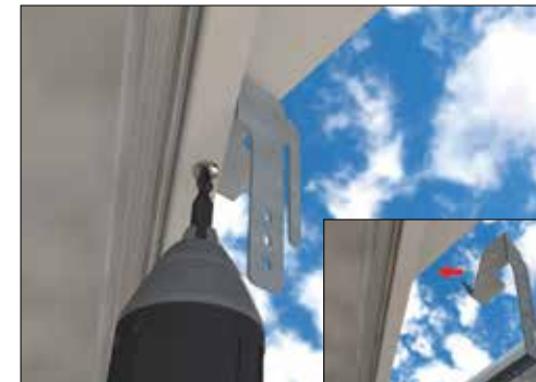
NOTE: The transom bracket CHA001 MUST be trimmed and adapted to suit situations where a transom bar, valley and pelmet vertical frame intercept, as shown above.
